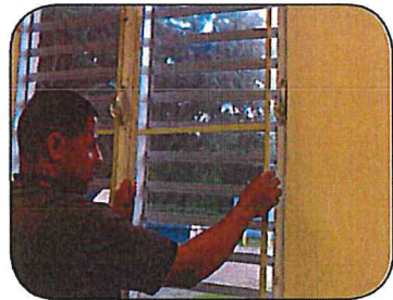
Install or repair window & door screens.
