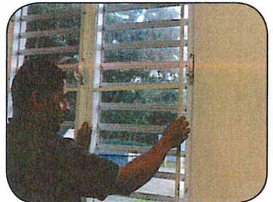
Install or repair window & door screens.
